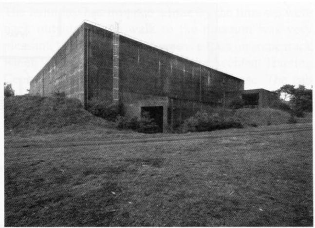
Avionics bunker. Photo: Nick Catford
